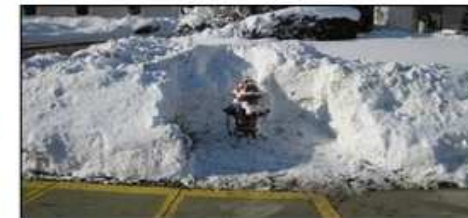
Photograph showing a properly uncovered fire hydrant (Source: MCFRS)
