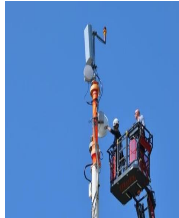
Installation of a mTBS
